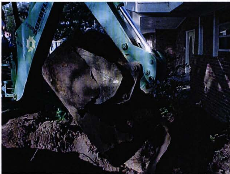
Laurel Bay #1 Tank One
