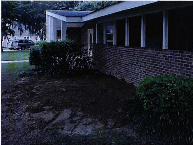
Laurel Bay #1 Post Excavtion
