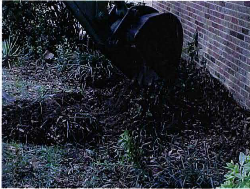
Laurel Bay # 1 Pre-Excavation
