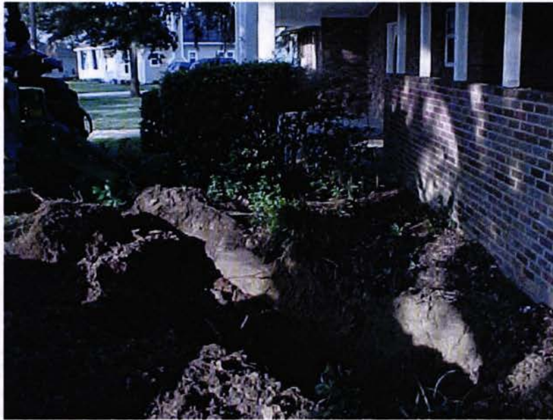
Laurel Bay #1 During Excavation
